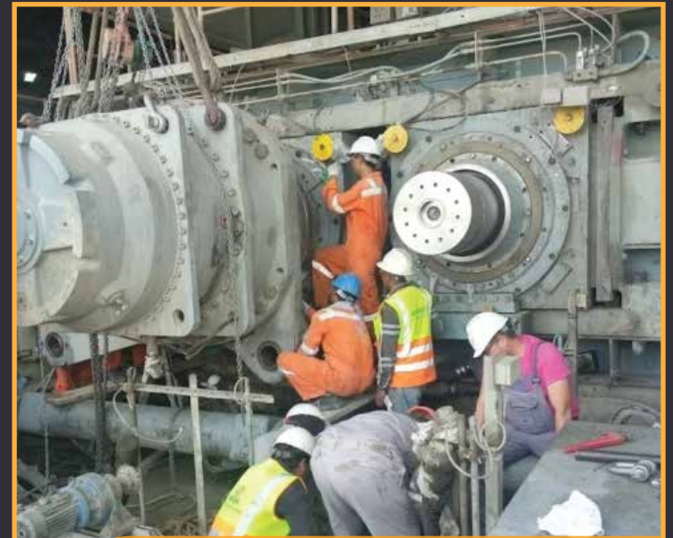
ROLLER PRESS MAINTENANCE SERVICES
