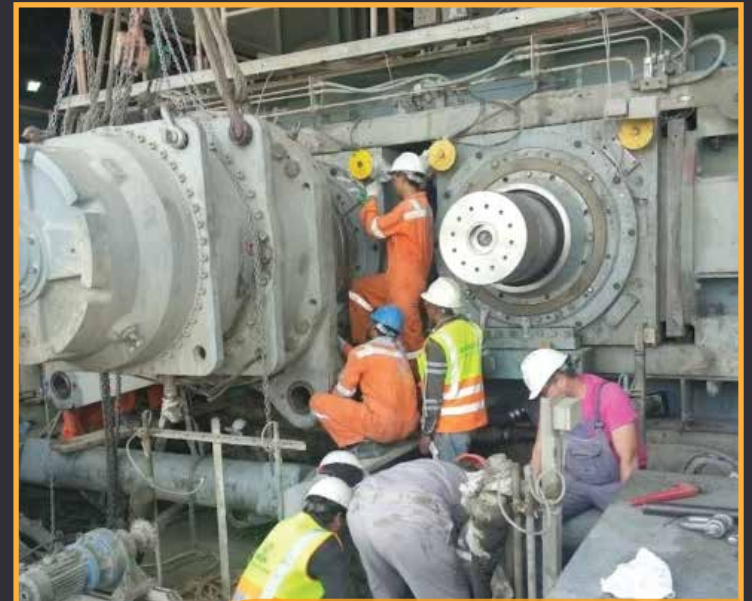
CM TRUNION REPLACEMENT
