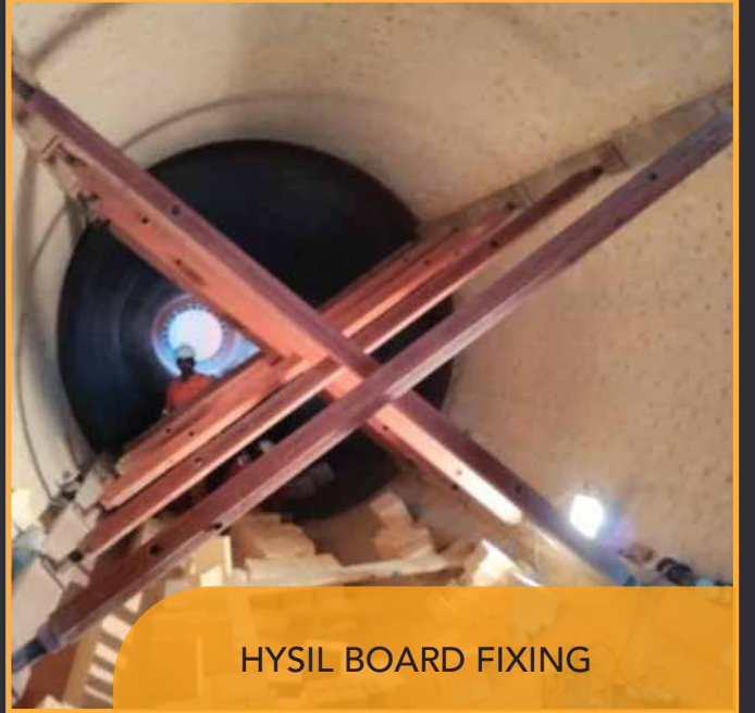
KILN HOOD REHABILITATION
