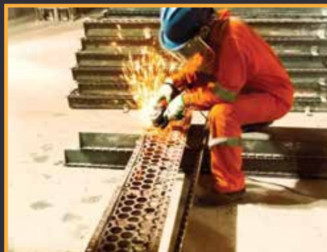
AIR SLIDE INSTALLATION
