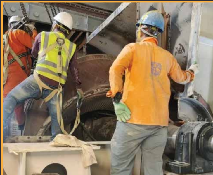
IMPELLER SHAFT REPLACEMENT
