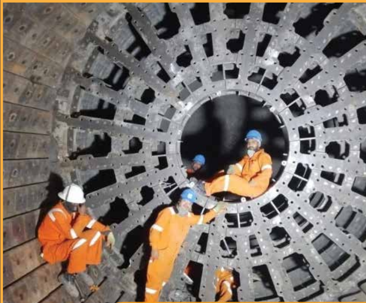
BALL MILL LINERS REPLACEMENT
