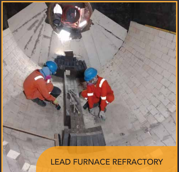
REFRACTORY BRICK DEMOLITION
