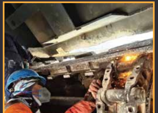
CRUSHER – APRON FEEDER OVERHAULING
